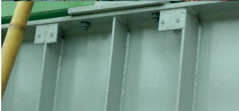
MTR 617- TKO South Station & Approach Structure 將軍澳南車站和引道結構
