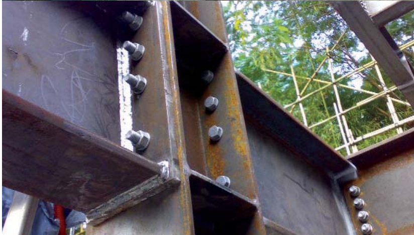
Customs Headquarters Building at North Point 北角電照街海關總部大樓
